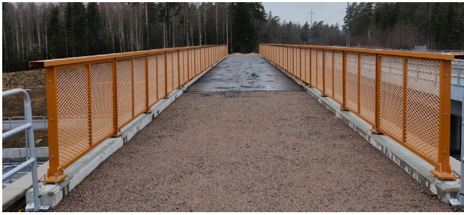
Fig. 4. The finished bridge with railings and asphalt.
