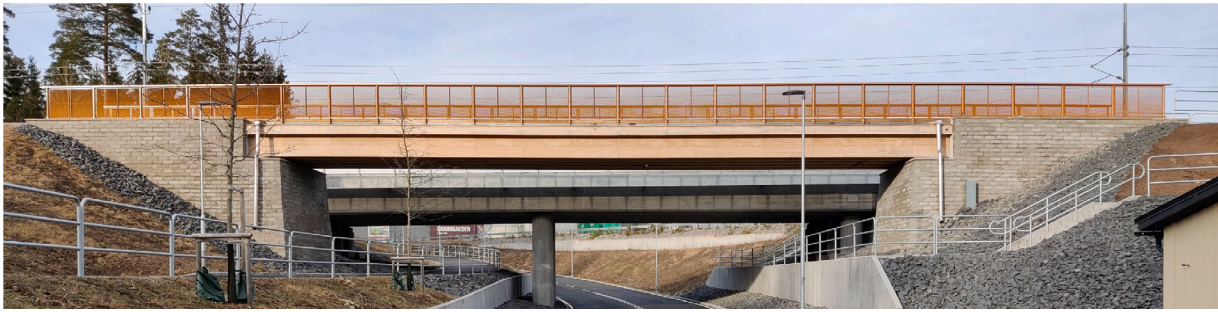
Fig. 1. The bridge viewed from the side.
