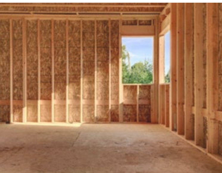
Lightweight timber frame with OSB sheathing
