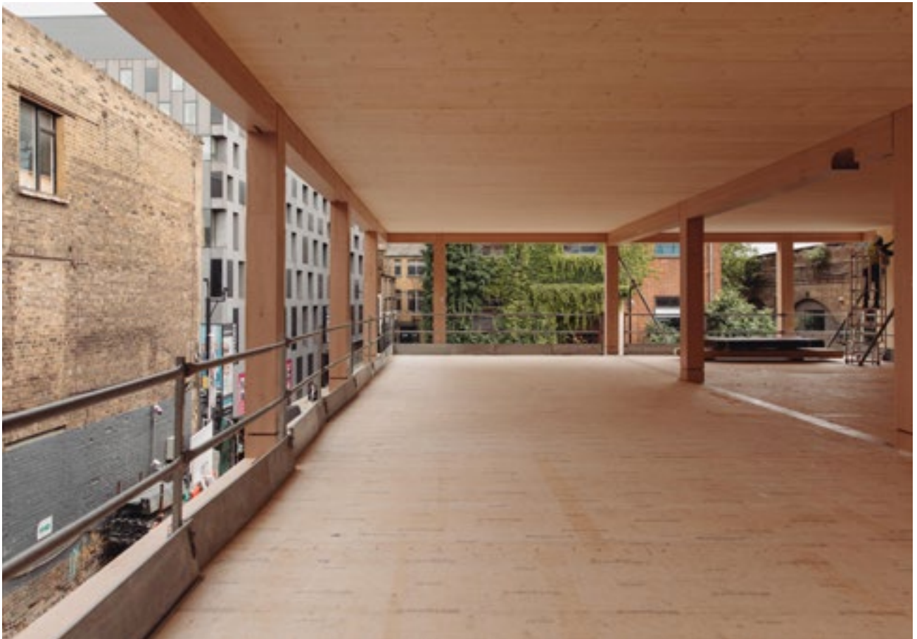
LVL post and beam frame in The Black & White building
