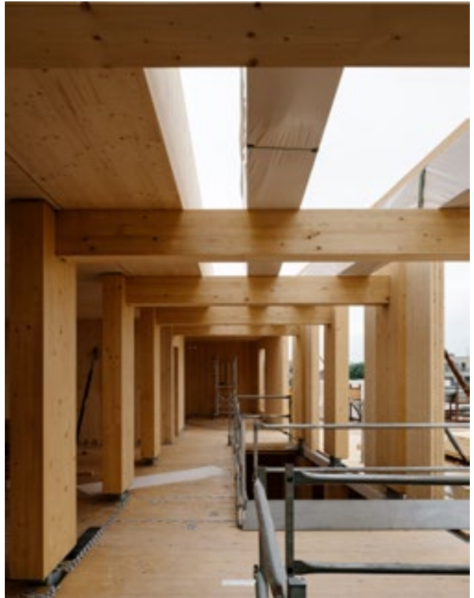
Glulam post and beam in The Greenhouse
