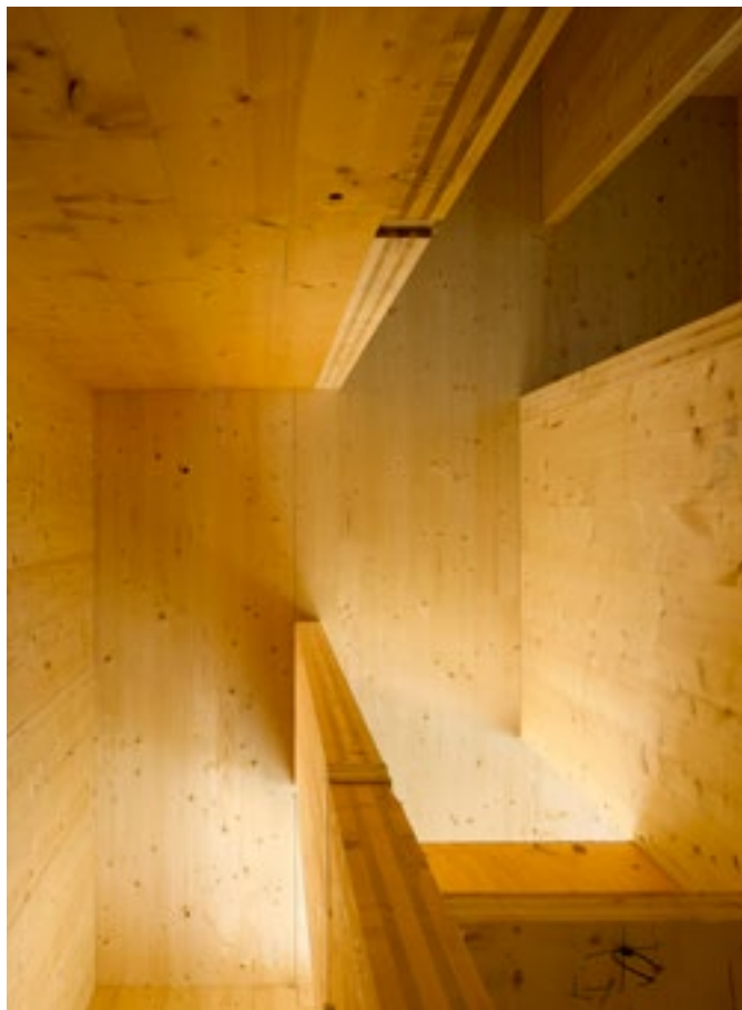
CLT walls and floors in Murray Grove
