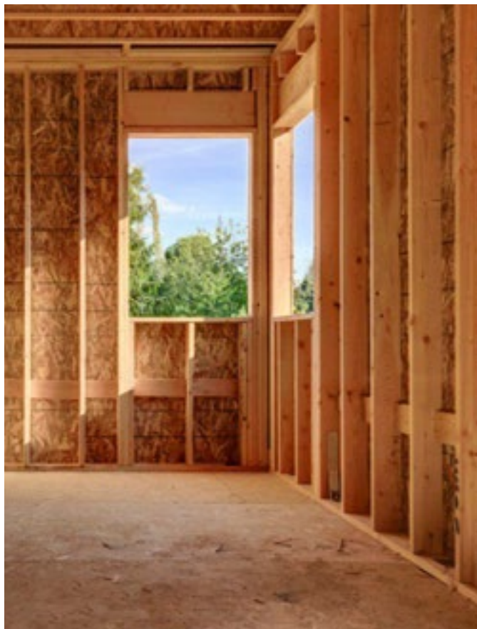
Open panel wall components in-situ
